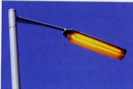
The distinctive shape and colour of SOX in action – but it could be a day burner
