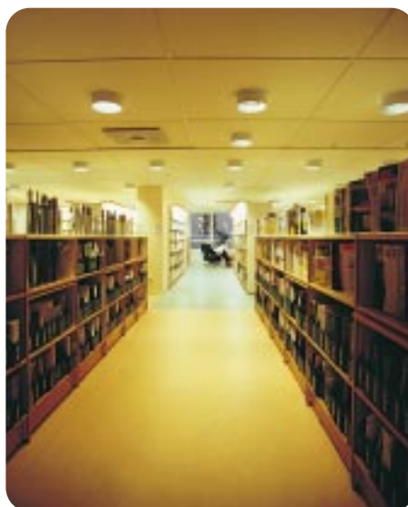
Energy-saving Biax downlighters replace incandescent lamps in this library.
