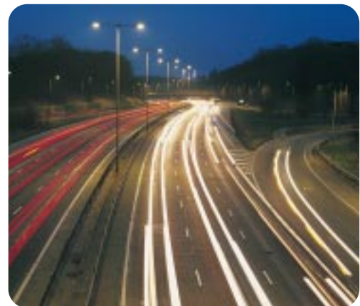
High Intensity Discharge lamps provide one of the most cost-effective ways of lighting public spaces.
