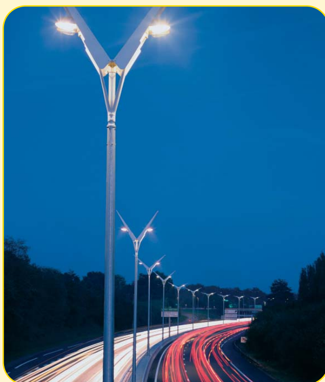
MASTER SON-T PIA - safe lighting for Bordeaux ring road
